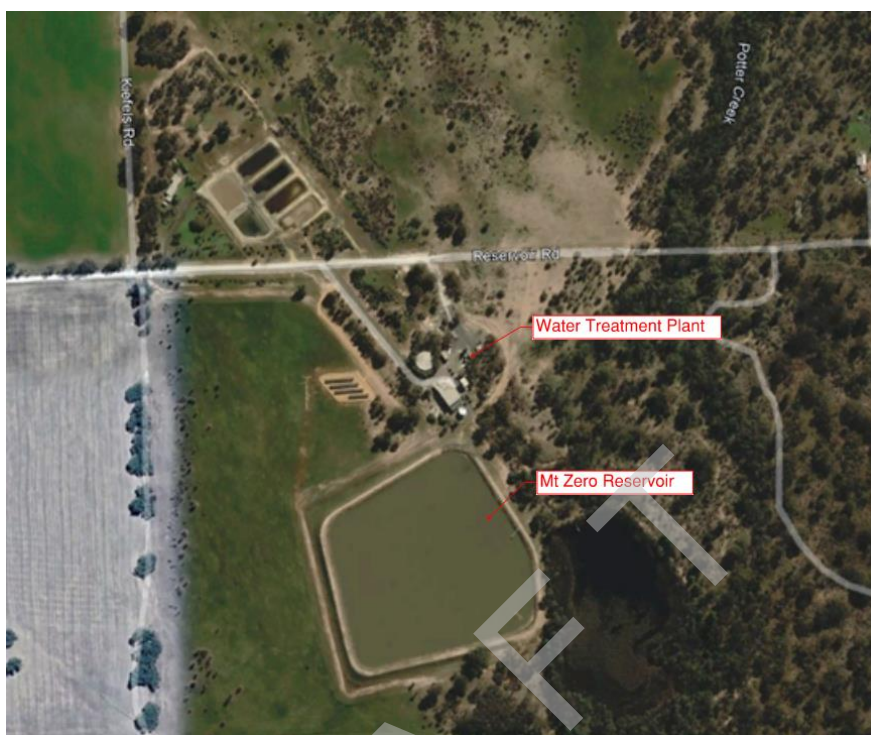
Figure 4 - Mt Zero Reservoir - Water Treatment Plant 5
