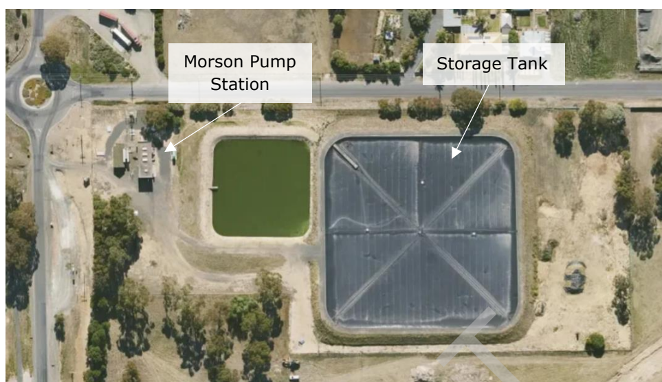
Figure 5 - Storage Tank – Morson Pump Station
