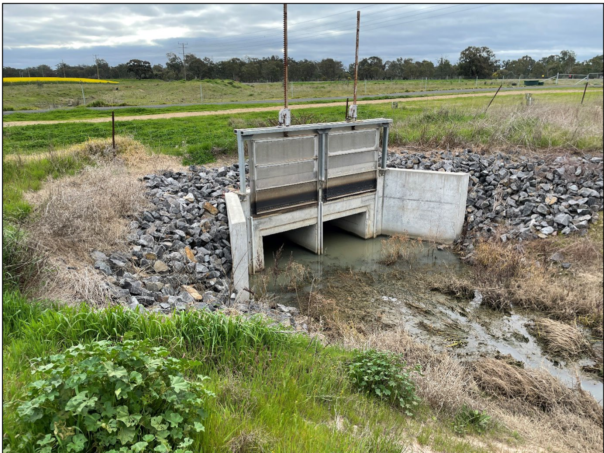
Figure 9 Existing outfall culverts at approx. 36.734S, 142.178E. Source: Site Visit
