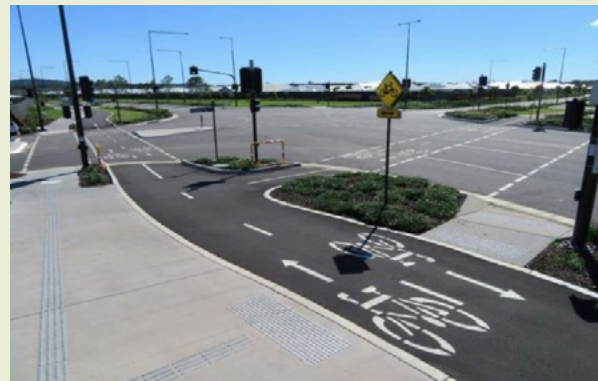
Treatment creating a protected intersection. Note the continuous cycle path and separation from pedestrians. Note also the landscaping barrier between vehicles and bicycles.
