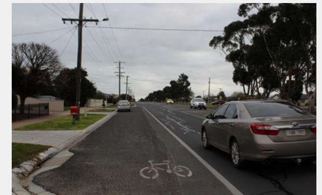
Natimuk Rd (looking west) – Cycle lane on arterial road not protected from high volume traffic.
