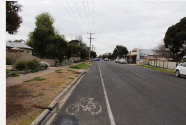
Bennett Rd looking north – Cycle lane on western side of road. Different width to lane on eastern side of the road.
