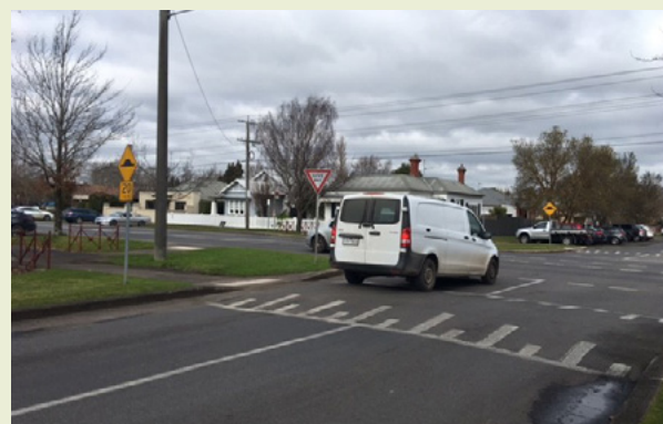
Speed calming treatment at intersection. (Ballarat, Victoria). Creates continuous pathway for cyclists and pedestrians crossing the intersection.
