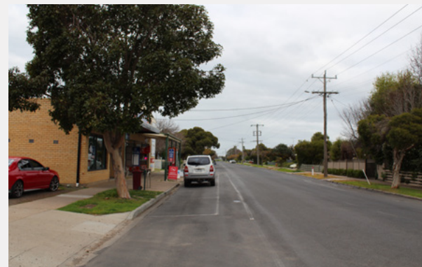
Bennett Rd (looking south) – Cycle lane gives way to parked vehicles.
