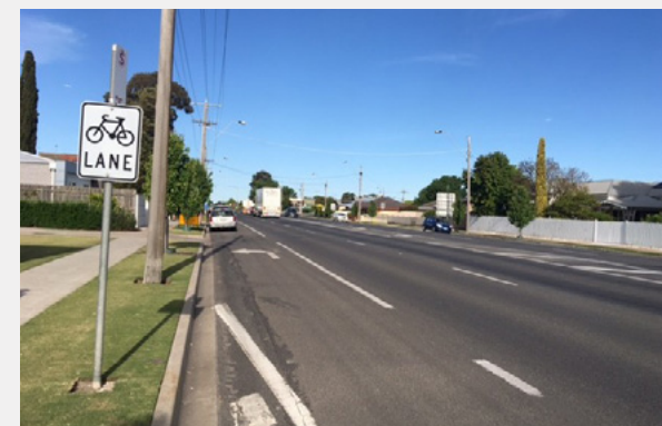
Baillie St (looking east) – High volume traffic and cycle lane is not protected and is shared with parked vehicles.
