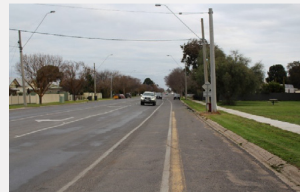
Cycle lane on arterial road not protected from high volume traffic.
