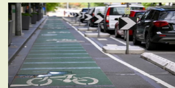
Protected cycle lane – Physical barrier and signage separates cycling from other road use.
