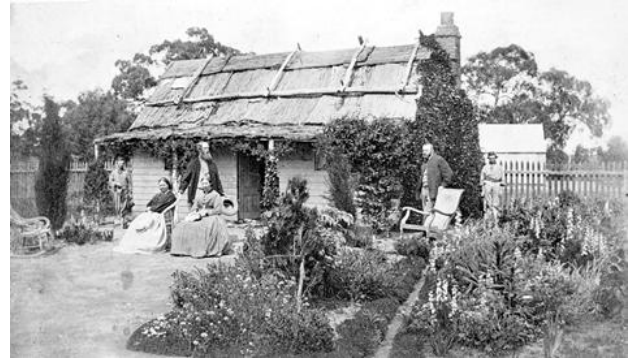
9.3 timber cottage at Green Park, near Horsham, with characteristic bark roof, c.1875 (Museum of Victoria)
