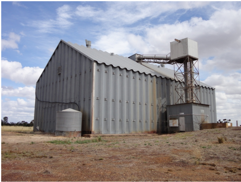
Behlen Grain Silo, 44 Noradjuha - Tooan East Road.
