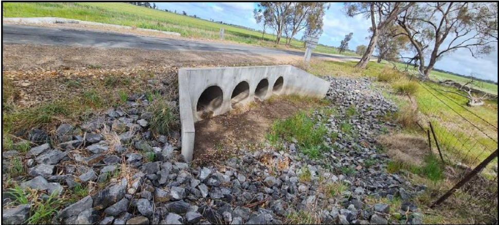
TYPICAL CULVERT CONDITION
