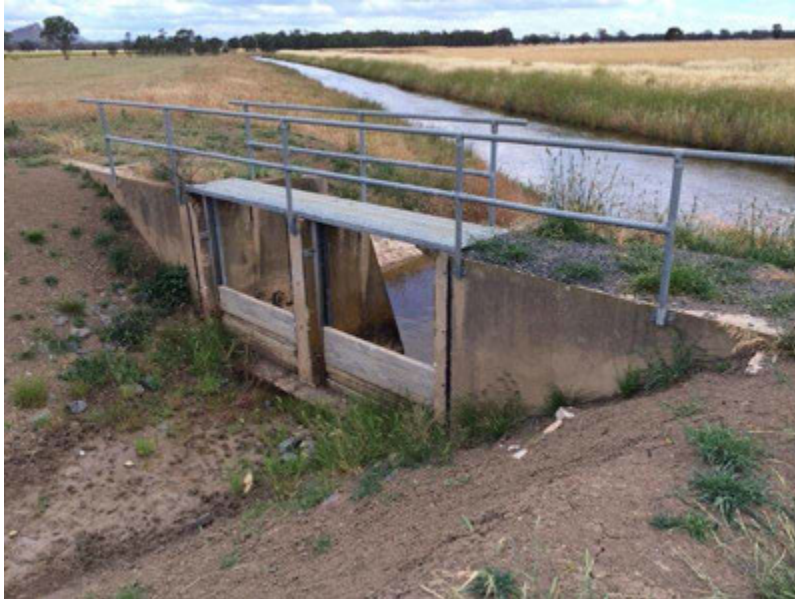
Wimmera Inlet Channel Loop Channel
