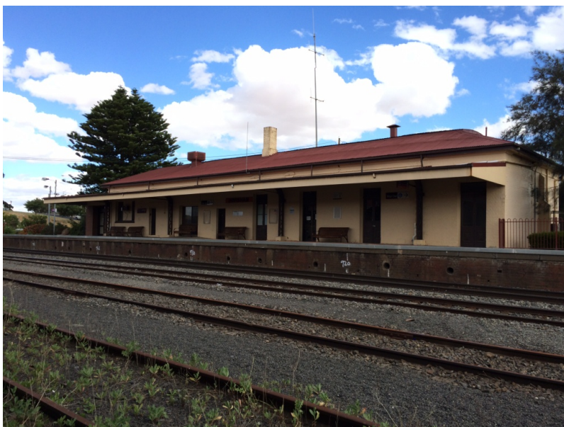
Horsham Railway Station, Railway Avenue Horsham
