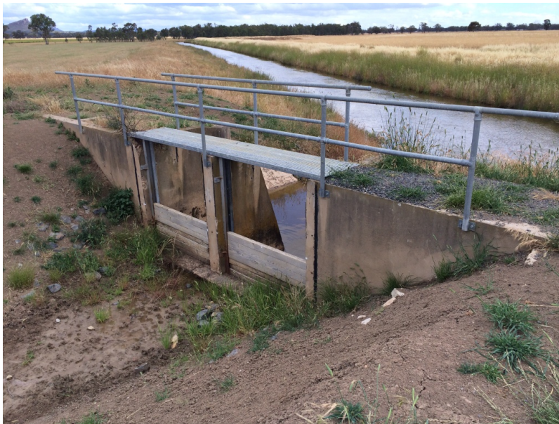
Wimmera Inlet Channel Loop Channel
