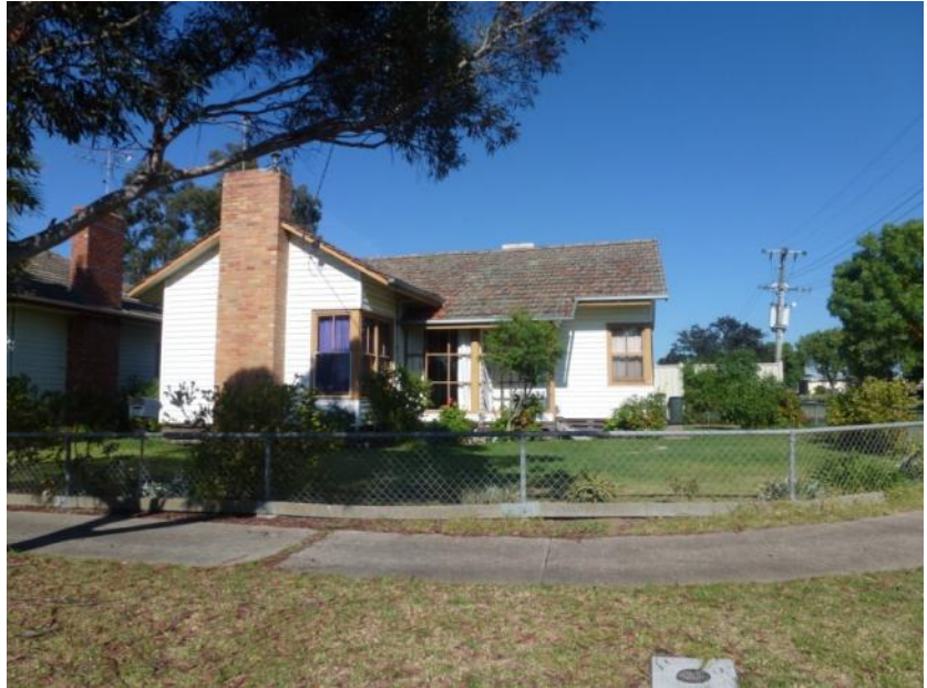
Typical 1950s Housing Commission dwelling, 2011, north Horsham
