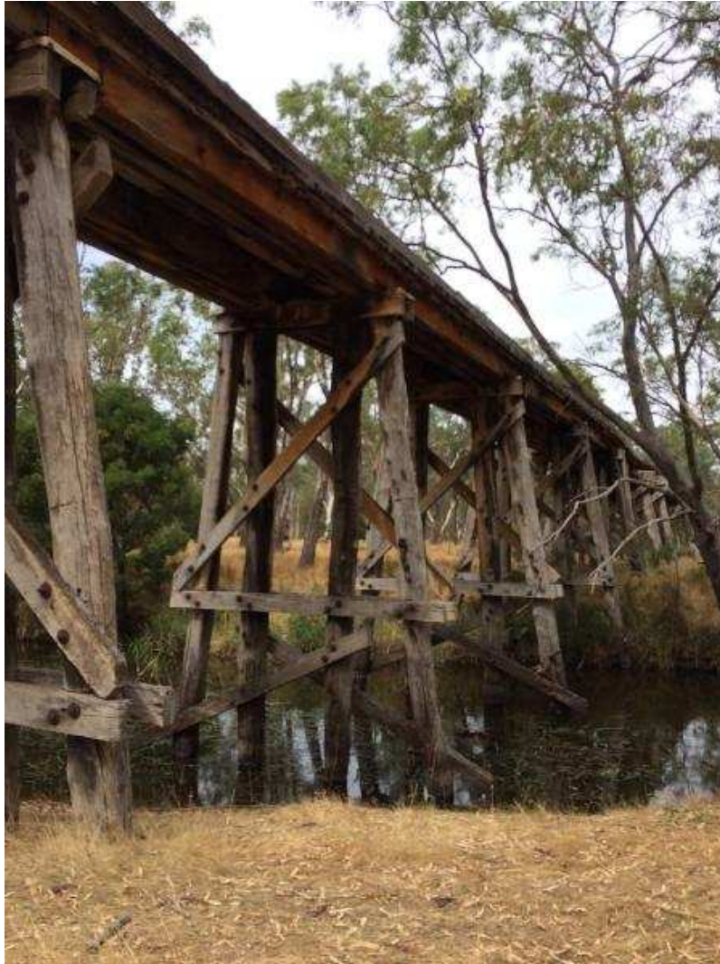
Timber Trestle Railway Bridge over Glenelg River
