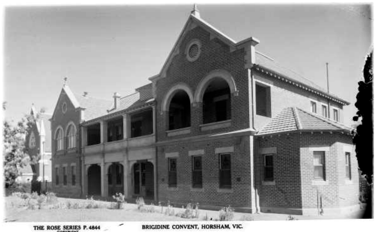
24.2 Brigidine Convent, Horsham, opened in 1920 – now demolished (State Library of Victoria)
