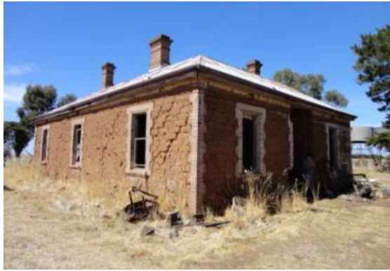
Oakville Park, Vectis c1900 mud brick homestead (2014)
