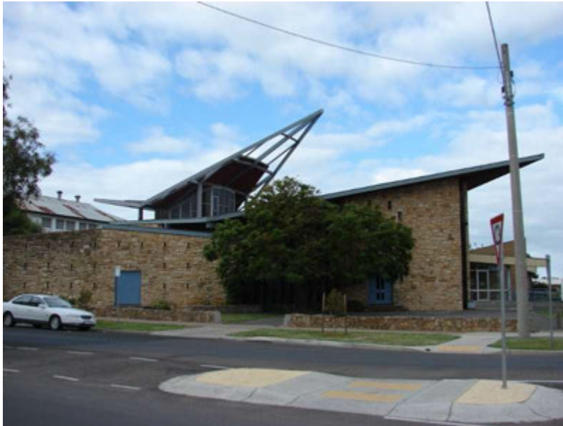
St Andrews Uniting Church, 8 Pynsent Street Horsham 141.JPG
