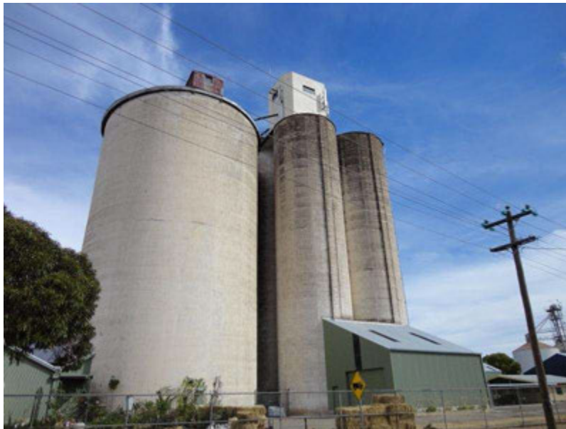
Horsham Silo complex, 35-39 Wawunna Road Horsham.jpg
