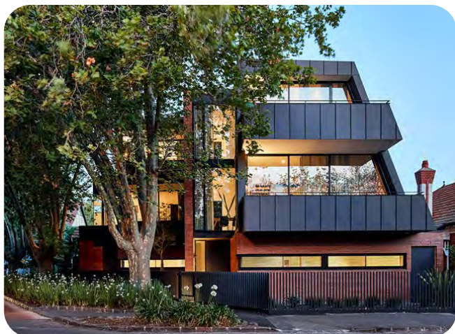
Contemporary street frontage and articulation
